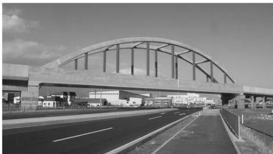
**Fig.1** Steel-concrete hybrid PC Langer bridge
