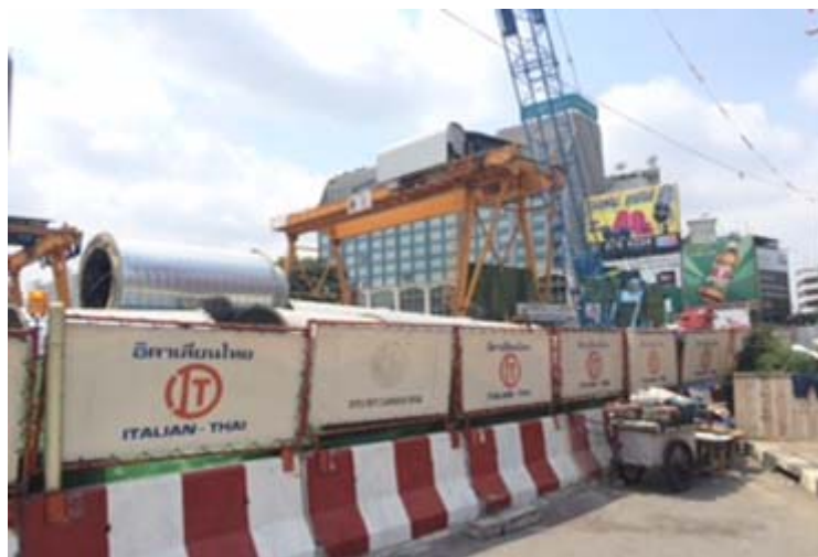
Technical Survey at Construction Site of MRT
