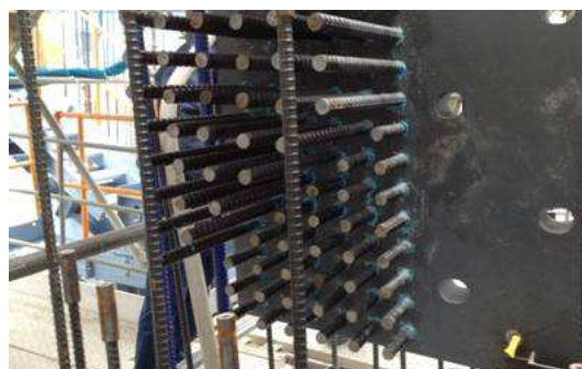
Fig.24-Re-Bar Connector
