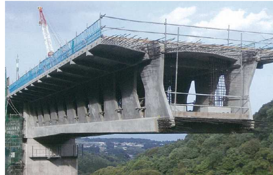
Fig.21-Butterfly Web Box Girder Bridge (Ashizuka et al., 2012)
