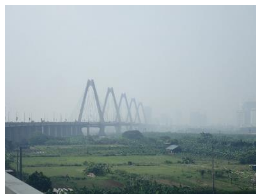
(4) Visit to Nhat Tan Bridge
